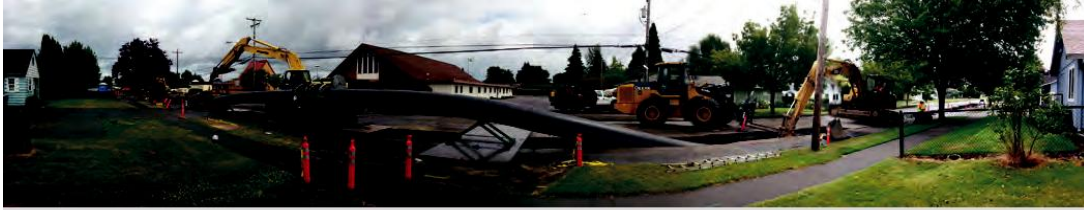
Water line construction on Hill Street.
