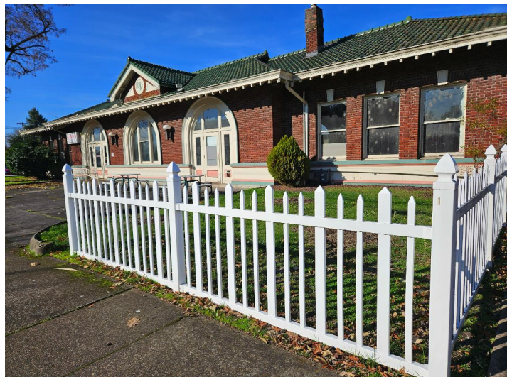
Exterior vinyl fencing to be removed.
