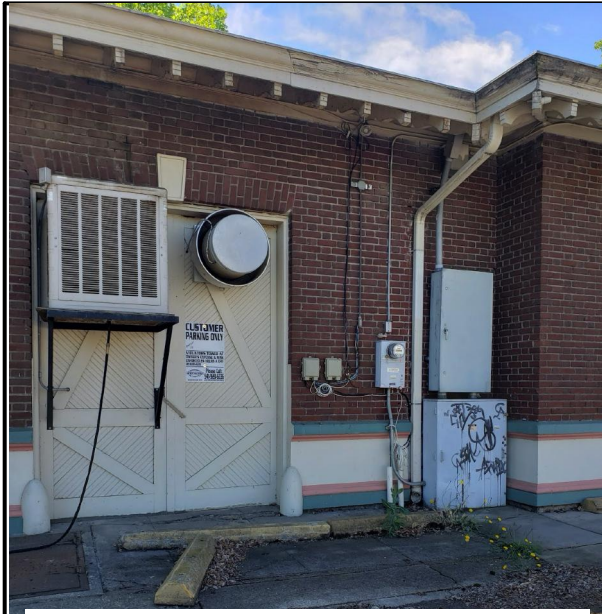
North exterior wall to become interior wall of new addition. Brick and other details to remain exposed on the interior.
