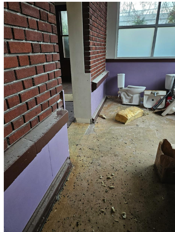
View of interior of annex connection. Existing walls to be restored when connection is removed.
