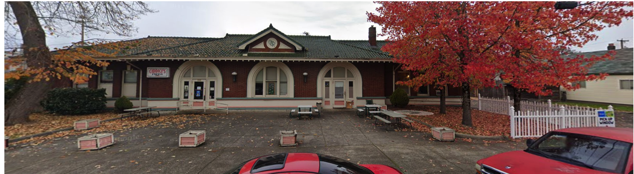
Existing south view of the train station.
