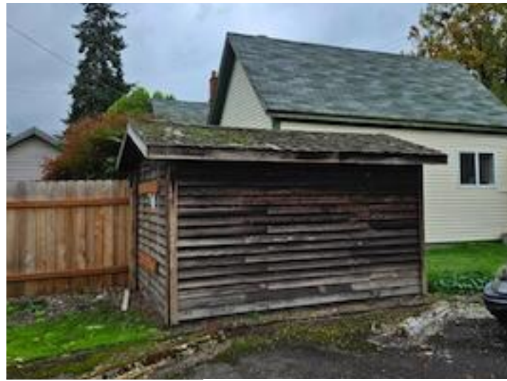
Shed to be removed.
