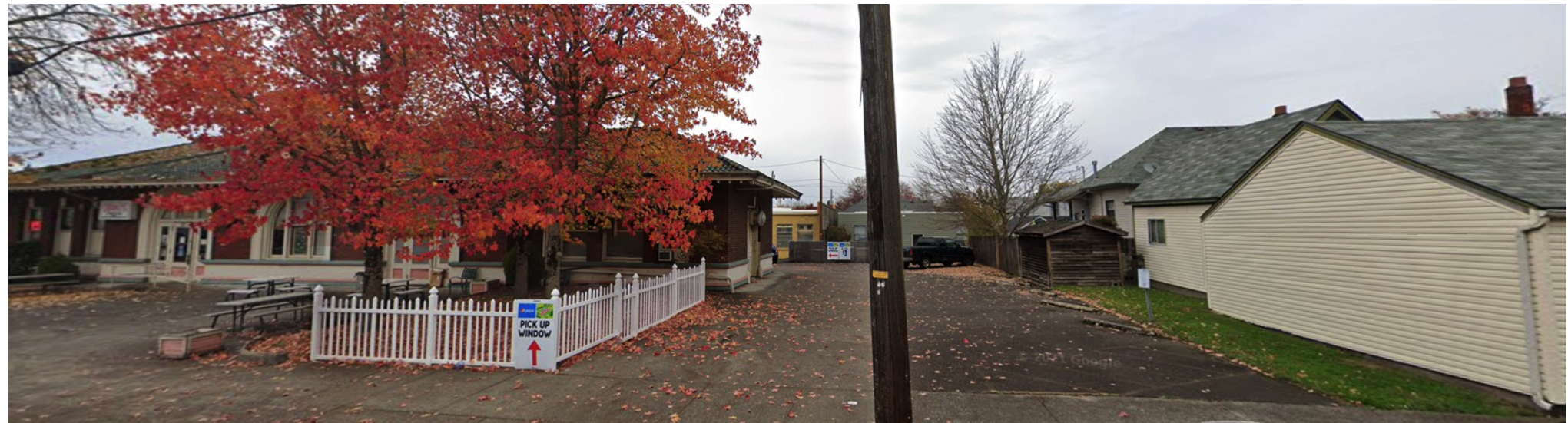
Existing view of where addition is proposed.
