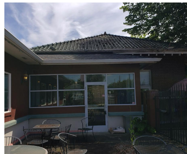
View of annex connection to be removed.
