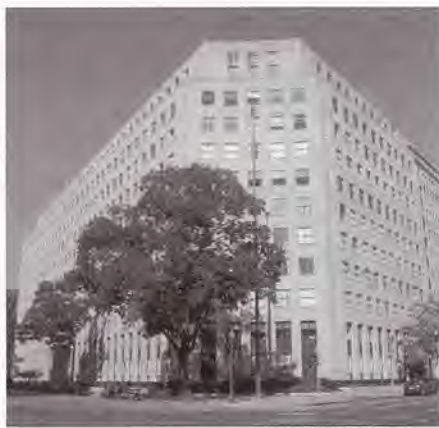
Fig. 1. Southwest elevation, Lafayette Building, Vermont Avenue and H Street NW, Washington, D.C. The building's neoclassical exterior has regularly placed, double-hung steel windows. All images by authors.
