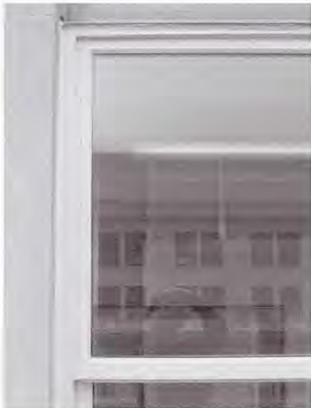
Fig. 6. Head of the replacement window.
