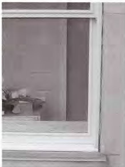
Fig. 5. Sill of the repaired window.
