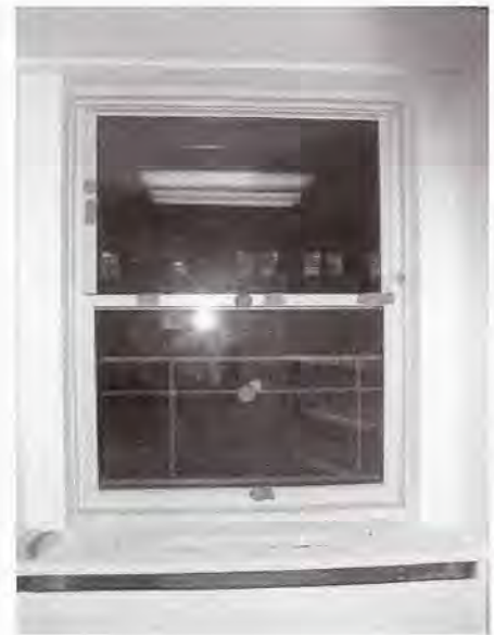
Fig. 9. View of the replacement-window mock-up prior to the installation of the interior chamber. The temperature sensors are indicated with dots.
