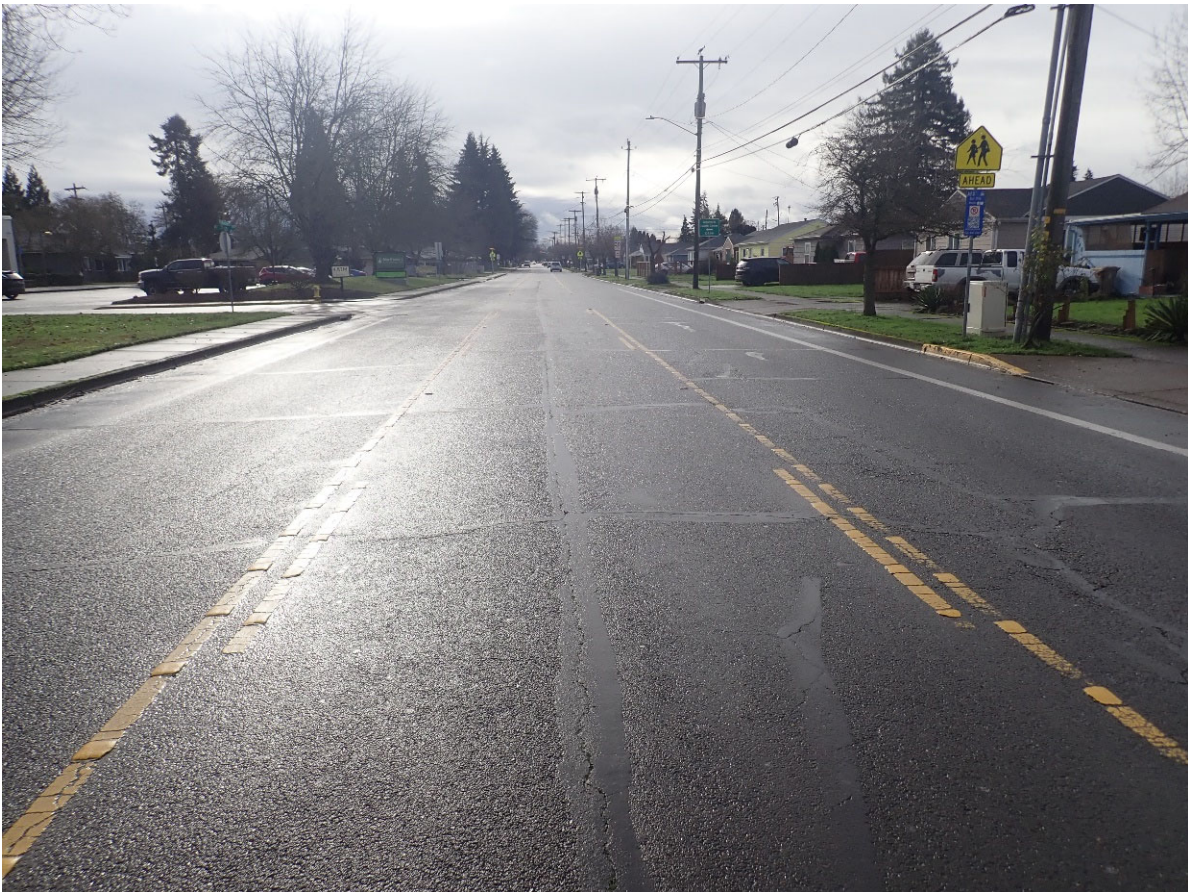
4. Looking northbound from 350 feet south of Albany-Junction City Hwy (99E).
