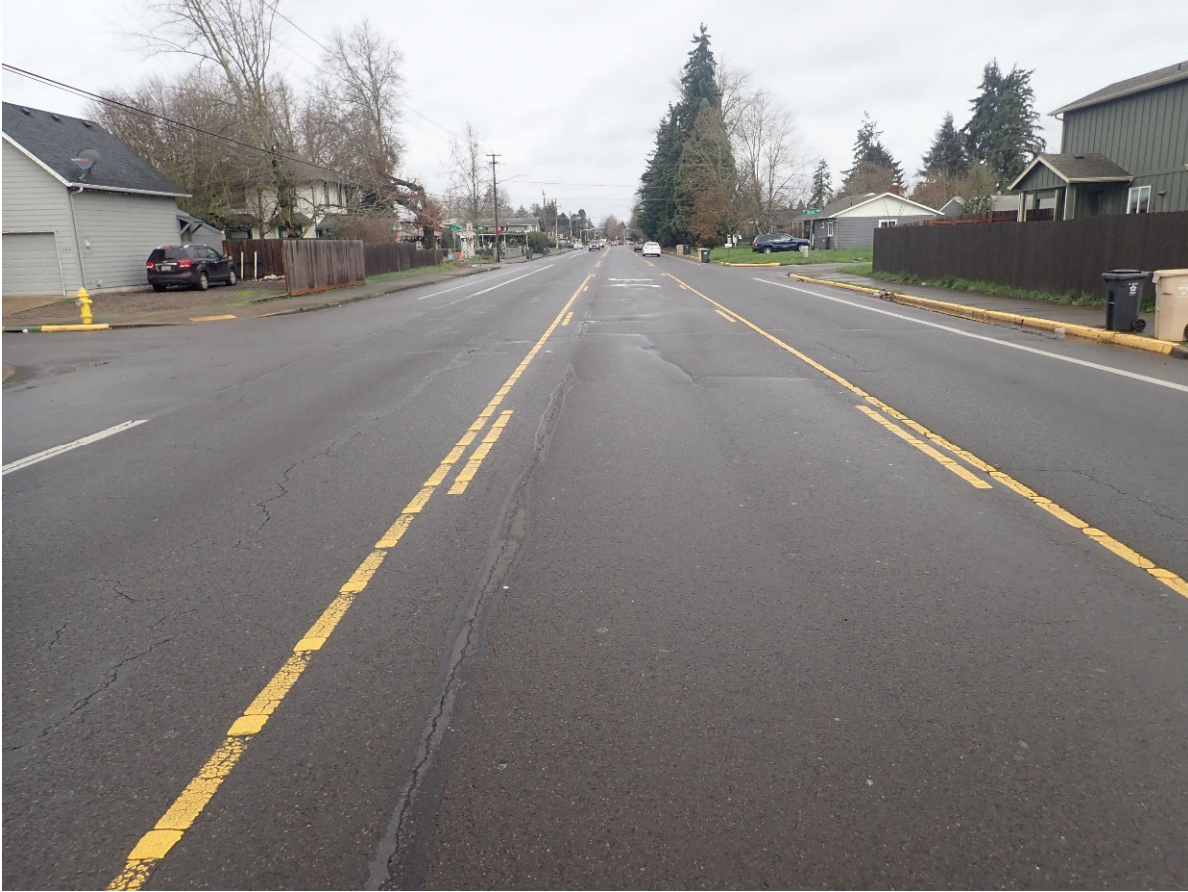
11. Looking northbound from 100 feet south of Waverly Court SE.
