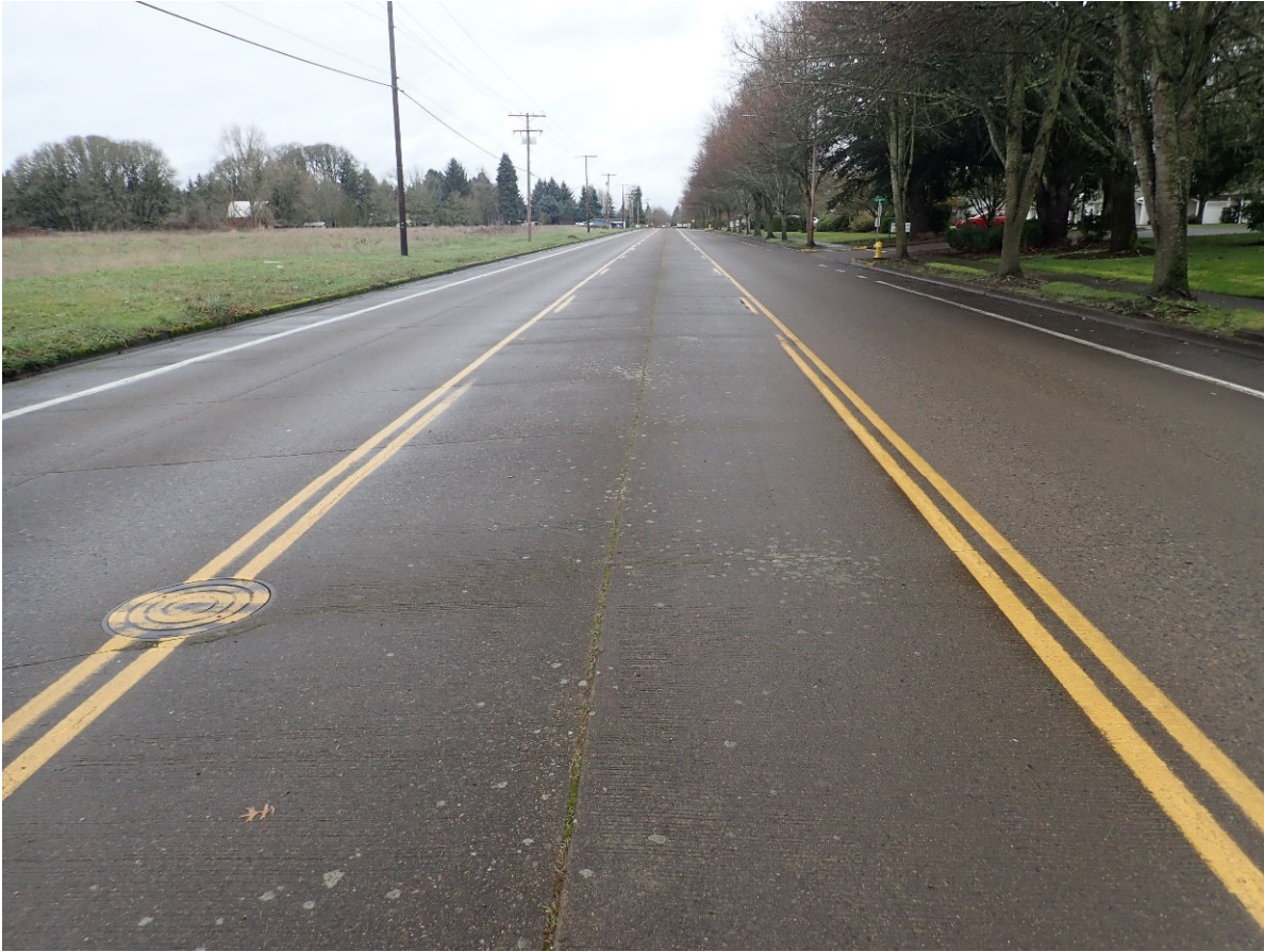
23. Looking northbound from 150 feet south of 54 th Avenue SE.
