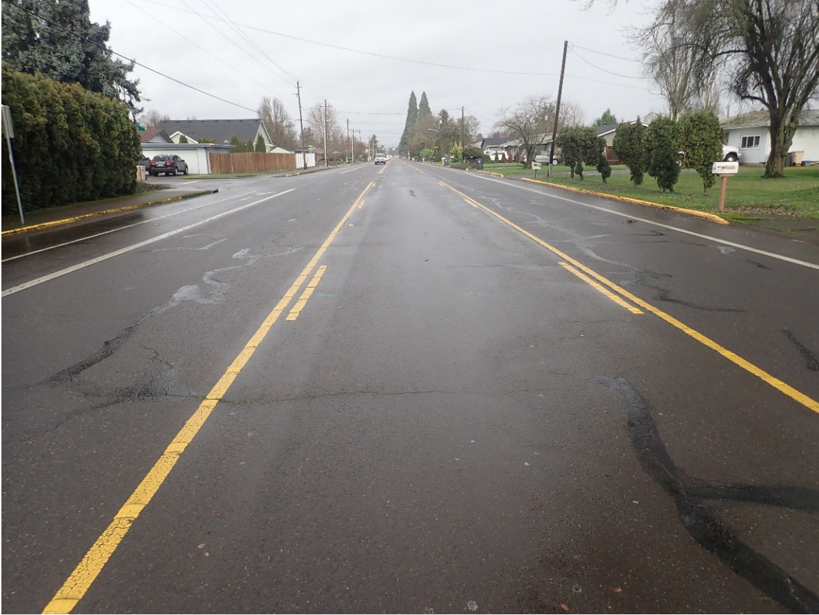
13. Looking northbound from 150 feet south of 25 th Avenue SE.
