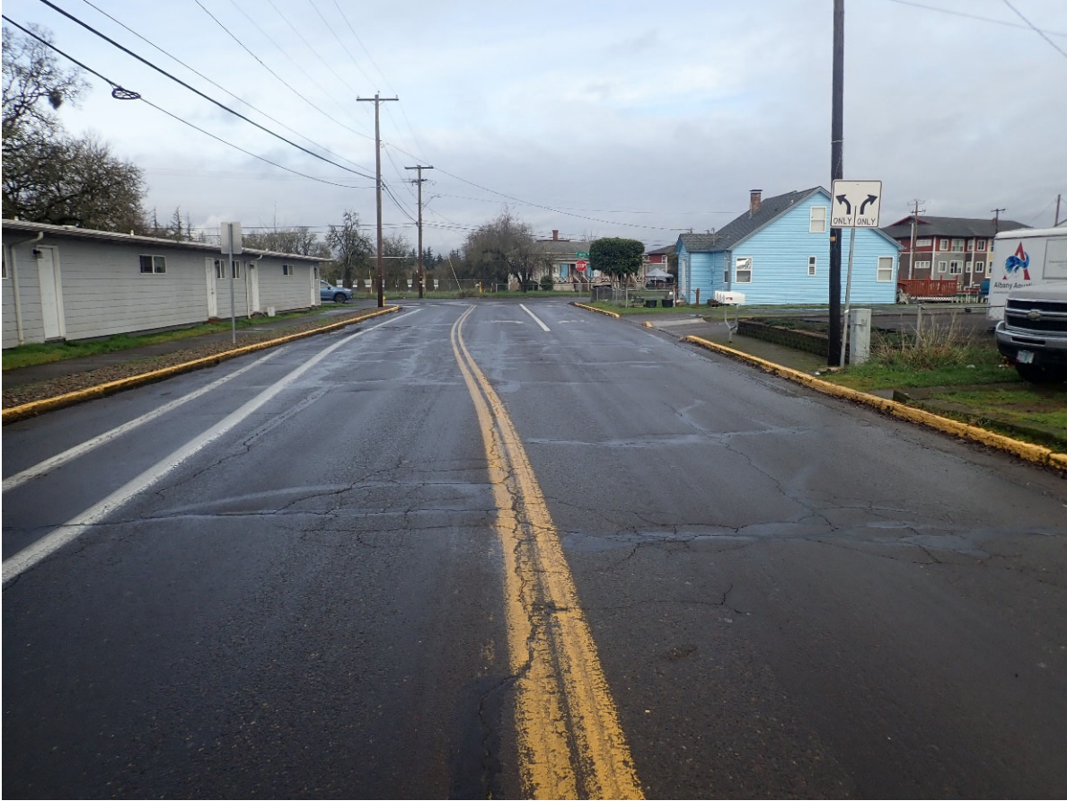
1. Looking northbound from 200 feet south of Salem Avenue SE.
