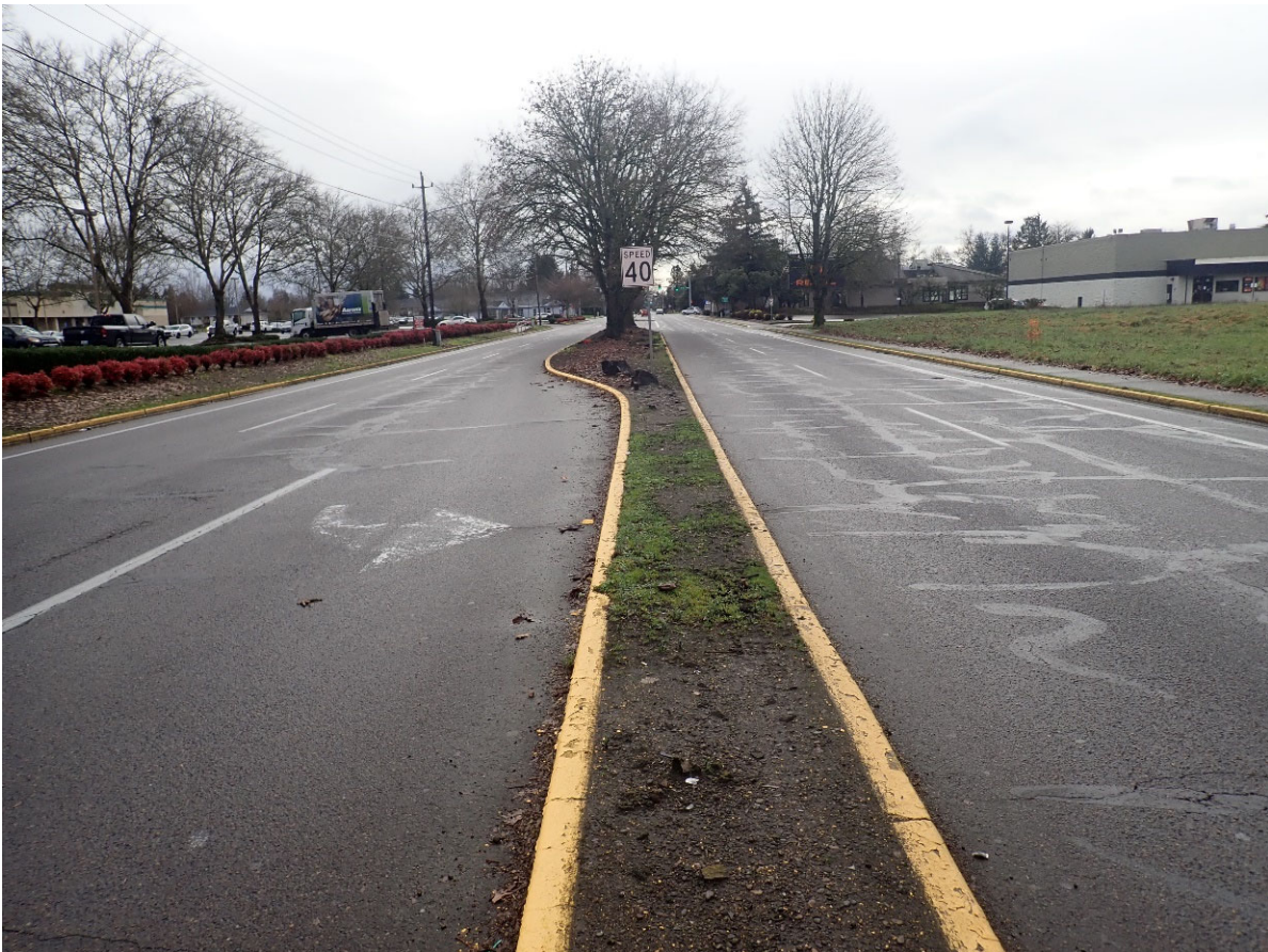
8. Looking southbound from 0.11 mile south of Santiam Highway (US 20).
