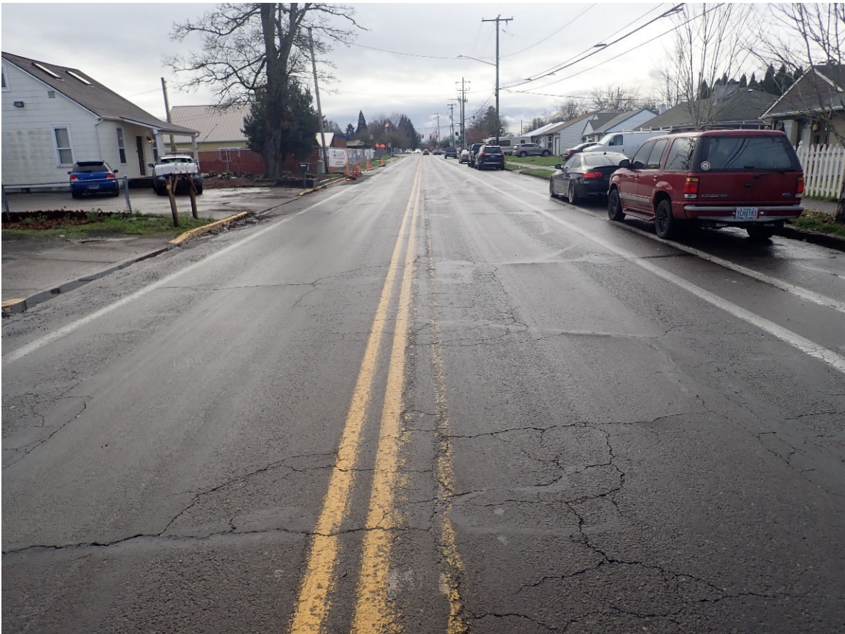
2. Looking southbound from 200 feet south of Salem Avenue SE.
