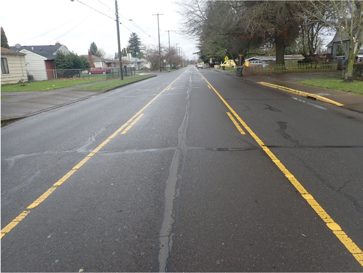
5. Looking northbound from 200 feet south of 9 th Avenue SE.
