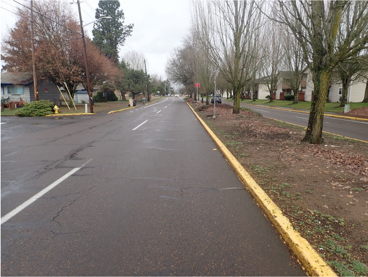
9. Looking northbound from 50 feet south of 16 th Avenue SE.
