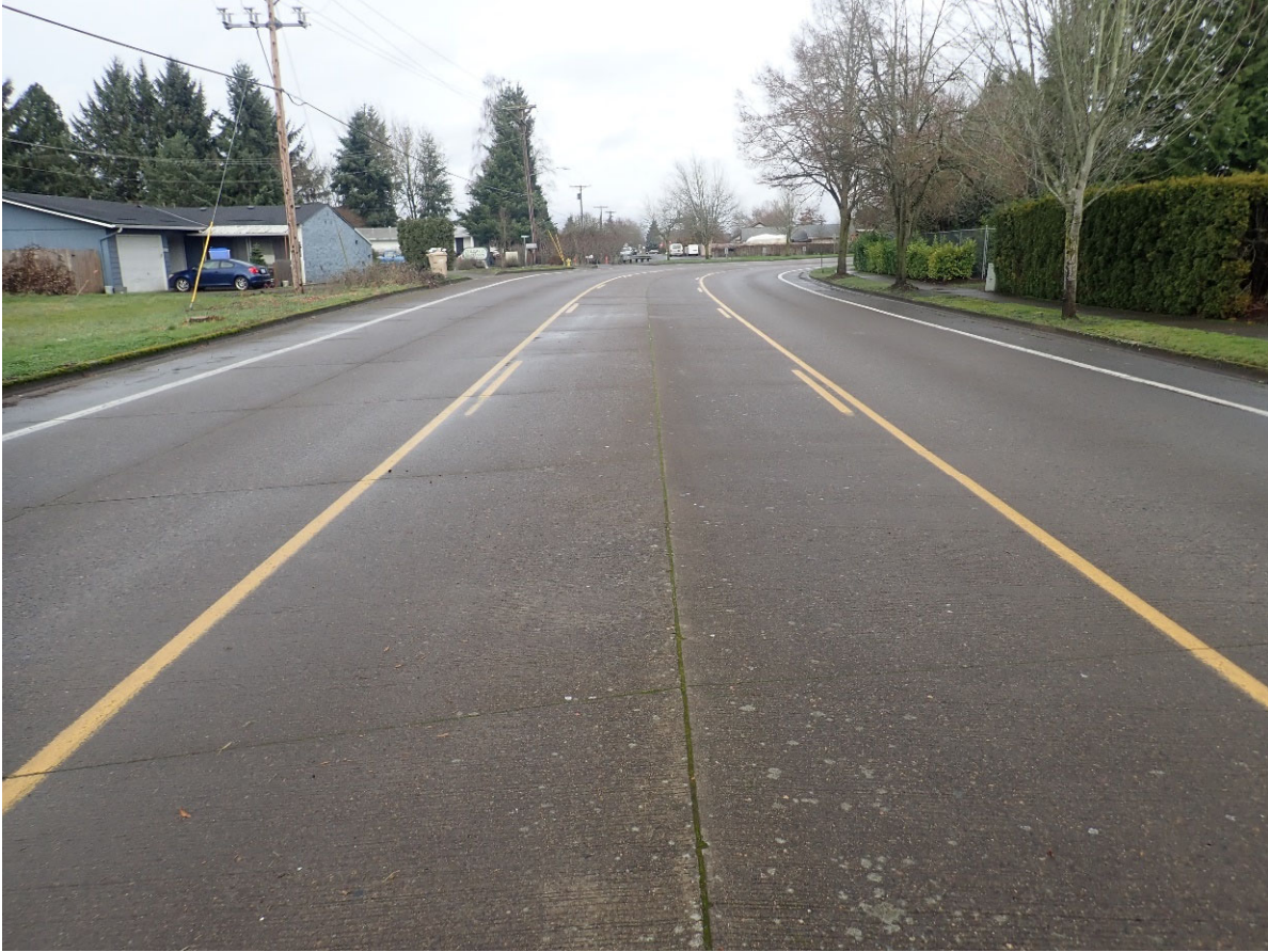
21. Looking northbound from 250 feet south of Cascade Drive.
