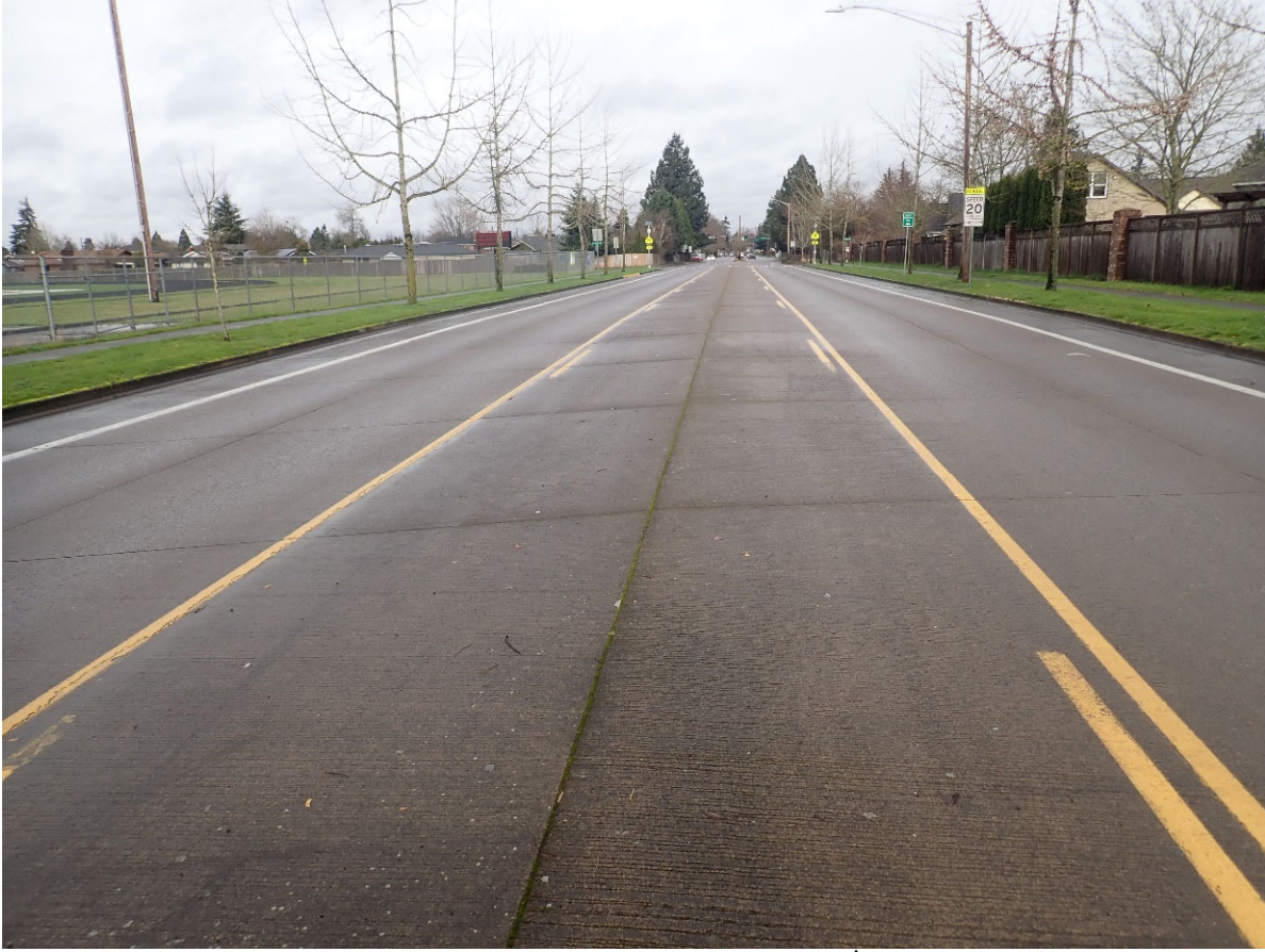
17. Looking northbound from 400 feet south of 36 th Avenue SE.
