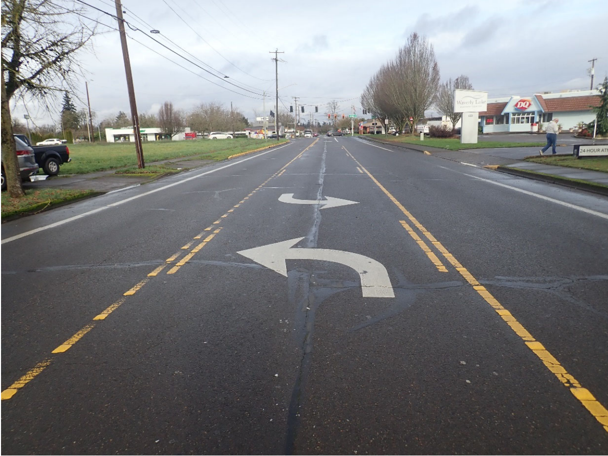
3. Looking northbound from 350 feet south of Albany-Junction City Hwy (99E).
