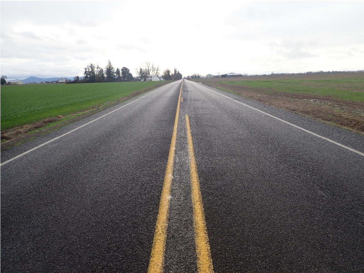
28. Looking southbound from 0.10 mile south of Ellingson Road SE.
