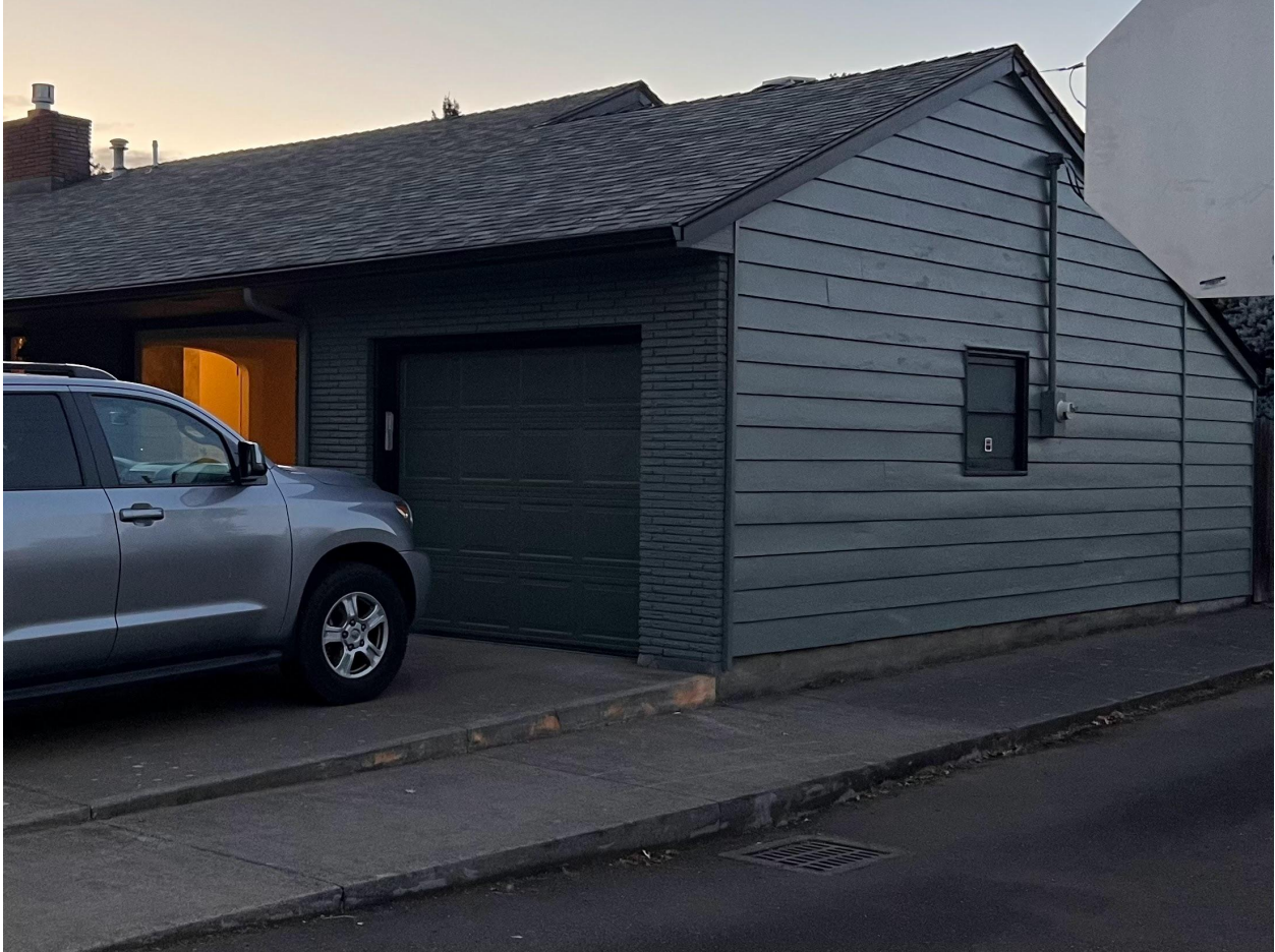
Combination of brick and vinyl siding - Corner of 5th and Vine
