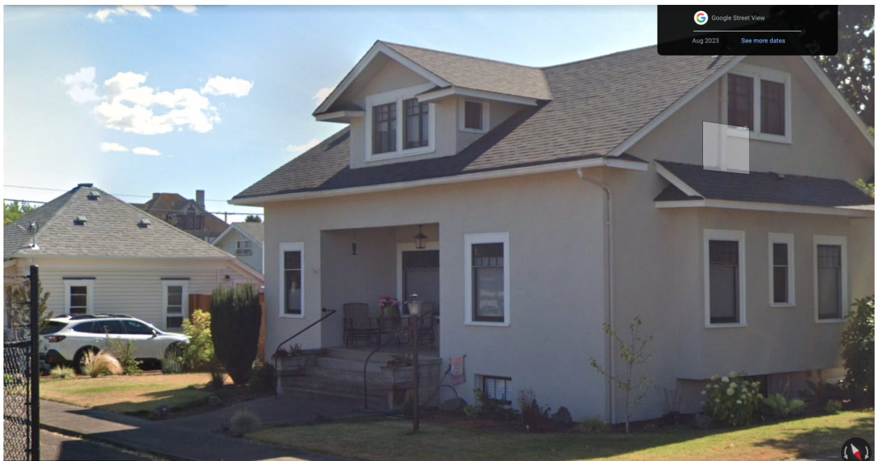
Stucco siding - corner of 4th and Vine
